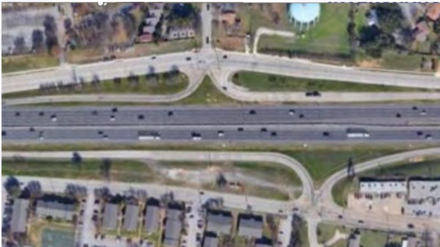
I-30 at Brick Street (Fort Worth, TX)
